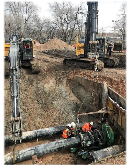
Crews fuse piping that has been installed under the Jordan River.
